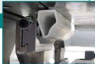
Fixing of glazing beads
